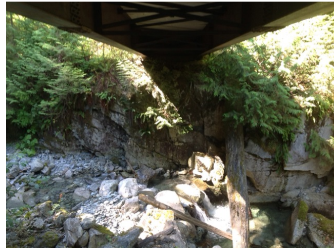
Left Bank Abutment when facing downstream
