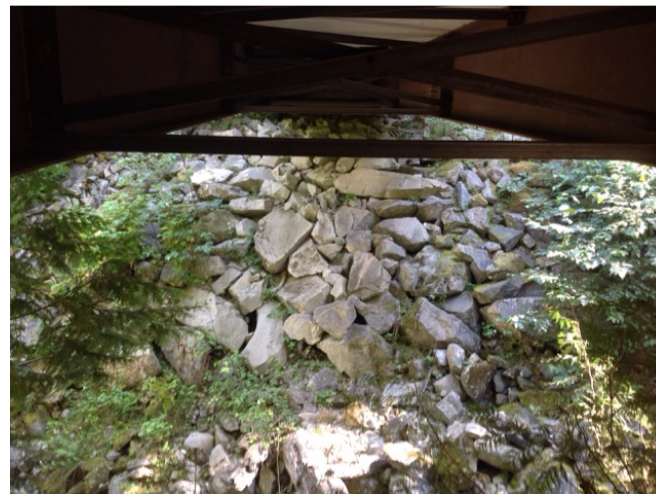
Right Bank Abutment when facing downstream
